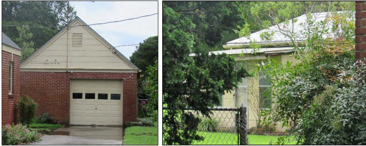
Photo 7: Garage, West Elevation (Left); Workshop Addition, North Elevation (Right).
