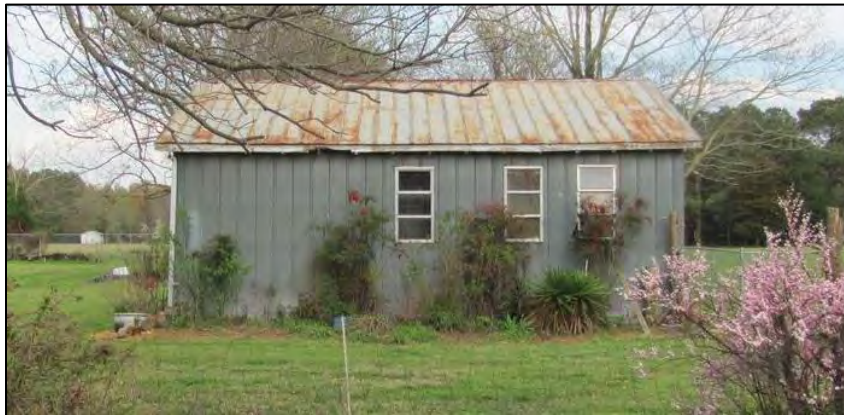
Photo 8: Shed, West Elevation. 19
