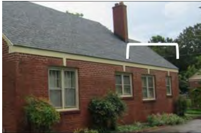
Photo 4: Rear Addition Noted in White, East Elevation.
