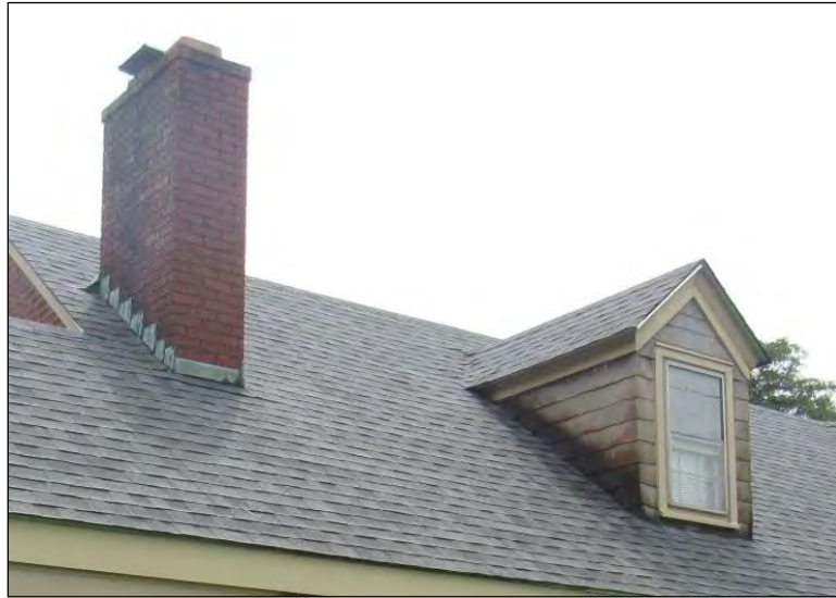
Photo 2: Detail of Dormer and Chimney Along Western Roof Slope, Facing Southeast
